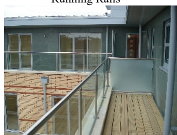
Sentinel with privacy screens
