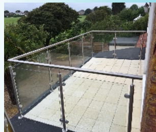
Glazed Sentinel to a balcony
