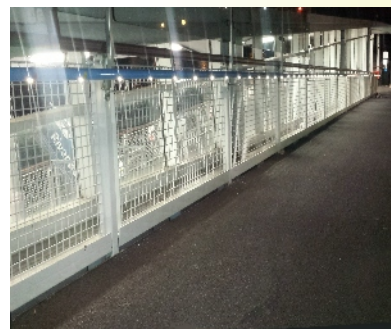
Illuminate-Stargard warm to the touch handrail with LED INSERTS
