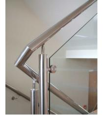
Handrail is either 42 mm or 48 mm diameter, and all "changes in direction" of the handrail are welded, dressed, ground smooth and then finally polished with either a bright or satin finish. We aim to have only one visible joint per flight of stairs.
