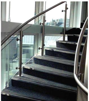
Various infills are available: Glass, perforated sheet, mesh, wire or "running rails."
