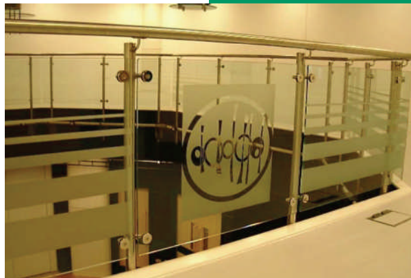
Balustrade with sandblasted logo and banding to the glass infill
