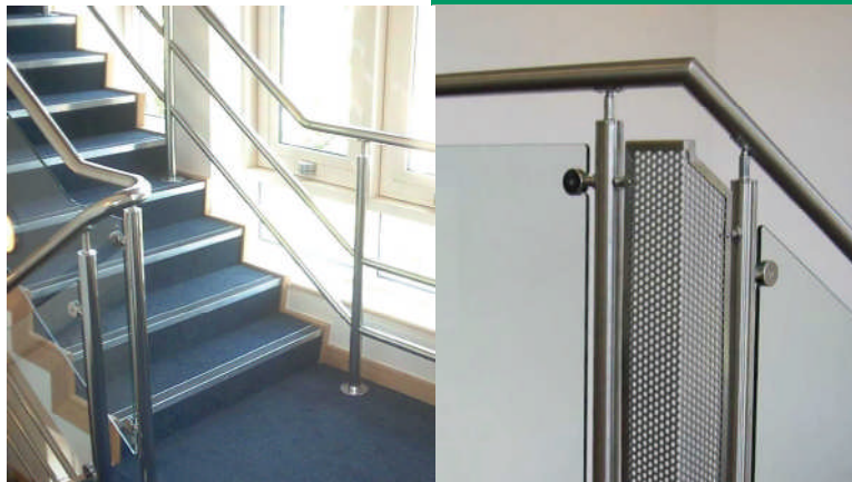
Balustrade with glass and mid rails
