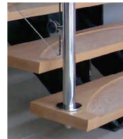
Wooden tread fixing
